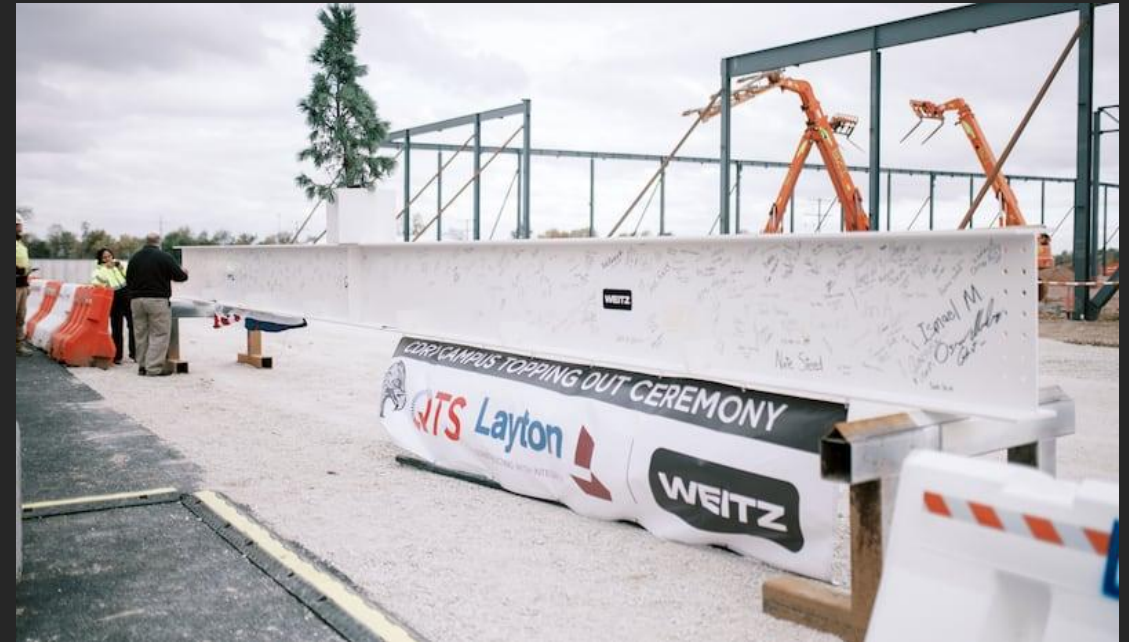
Cedar Rapids data center campus, topping out ceremony, Oct. 21 st , 2025
